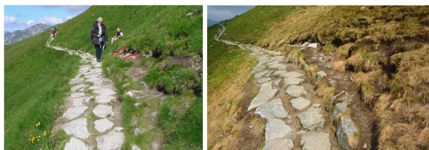
Widening of tourist path on sites no 3. The path is hardened and should be protected against erosion, but paths is too narrow
