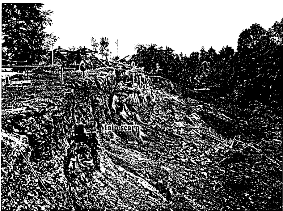
Photo 2. Landslide in Falkowa, July 2001
