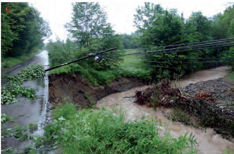
occurred in the Lanckorona commune over a period of four days (17–20 May), causing significant damage to housing and technical infrastructure. The landslides occurred mainly due to the clay cover and the underlying layer of loam, loose rocks, and interbedded slate with sandstone being saturated with water (Bajgier-Kowalska 2011).
