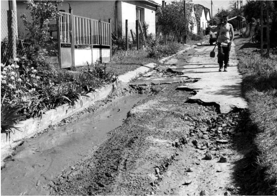
Photo 4. Erosion by flash flood in Nagykónyi. Street pavement was washed away (Photo by Sz. A. Fábián)
