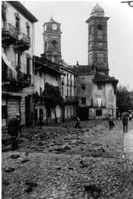
Fig. 8. The presently-called "Piazza Molines" (Giaveno), flooded by muddy debris rushed out the Rio Botetto culvert underlying a closely-driving street on September 1949 (Courtesy Lions Club Giaveno)
