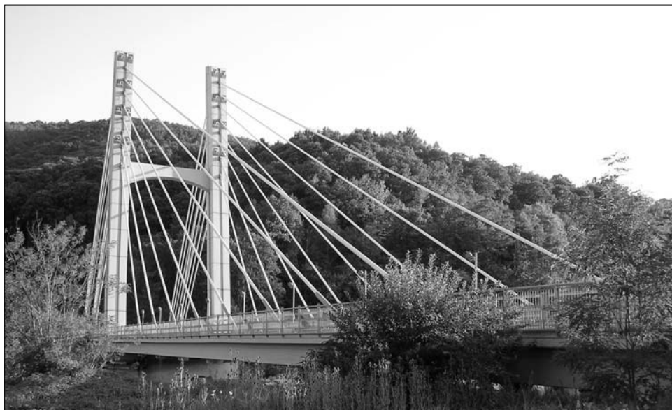
Fig. 3. The “Cumiana” bridge on the Sangone torrent, along the provincial road No. 193, was re-built after the old one collapsed during the October 2000 flood. From the end of the 19 th century onward, such artifact was damaged and reconstructed at least three times: in the 1890s in concrete blocks, in the 1950s through reinforced concrete and recently (2002–2005) in a cable stay structure. The recently-built artifact is more than 15 m long; piers are found along the right bank
