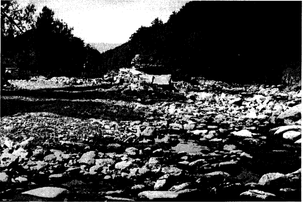
Photo 4. Pillar of a destroyed bridge on Wilczka river, where major avulsion took place (by R. Żurawek)
