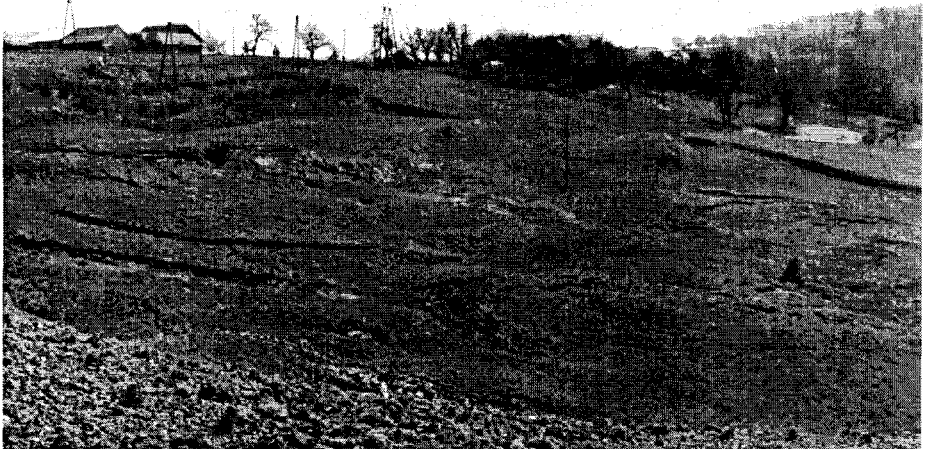
Photo 7. Landslide in Szczepanowice, gmina Pleśna (17 April 2000)
