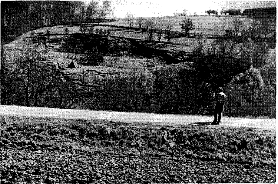
Photo 6. Landslide slope in Rychwałd, gmina Pleśna (17 April 2000)
